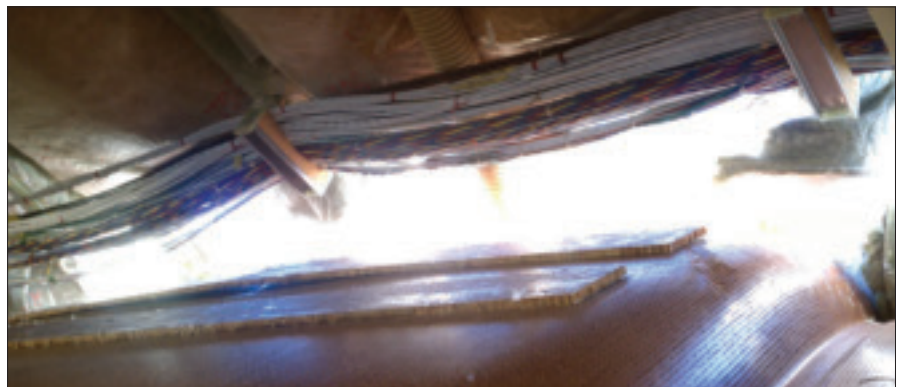
On April 1 a 5-ft hole opened in the roof of a Southwest Airlines Boeing 737-300 on its way to Sacramento.
